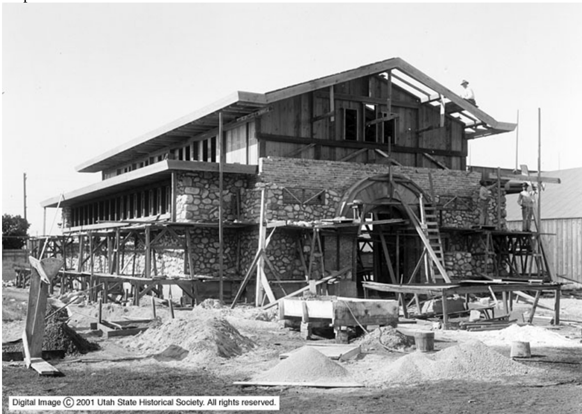
Construction of the Wildlife Building at the Utah State Fairpark
